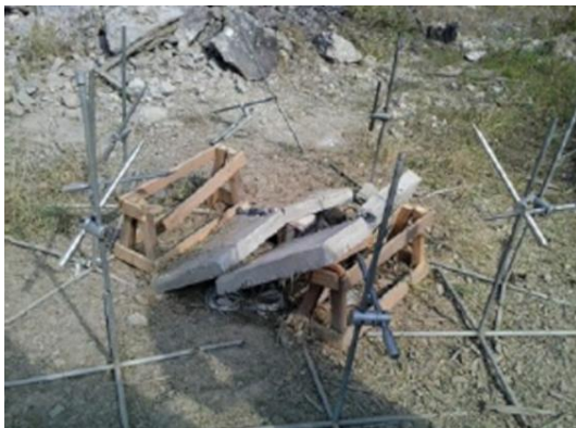
Fig. 1. Slab 1 after explosion [20].
