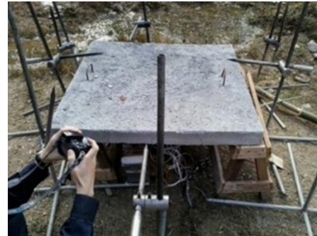
Fig. 2. Slab 6 after explosion [20].
